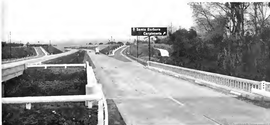
Looking west. Carpinteria Creek Bridge in foreground and on-and off-ramps for Carpinteria connecting to Casitas Pass Bridge.
